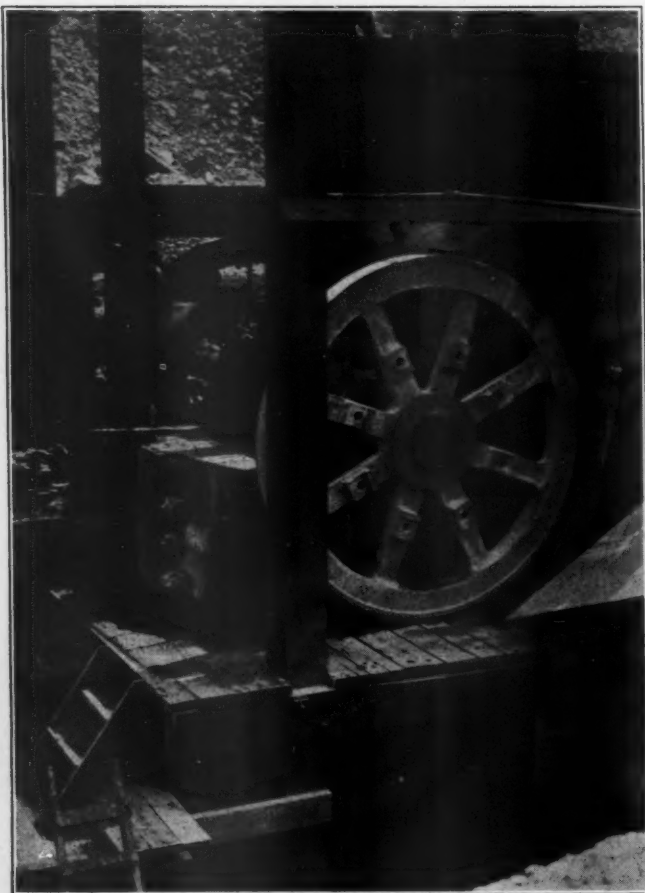
Rear View of the Primary Crusher
